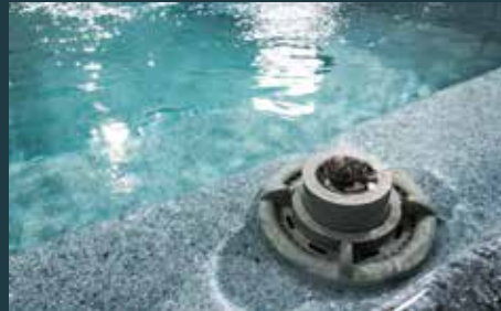
INTEGRATED SKIMMER For cleaning the water surface
