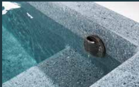
SAFETY OVERFLOW Protects the pool against overflowing in the event of heavy precipitation
